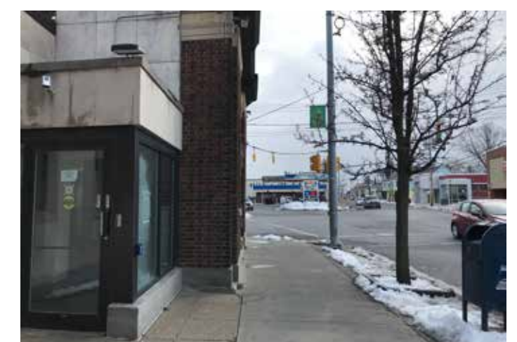
Some portions of the sidewalk have pavement that is in relatively good condition and there are a few street trees along the corridor to the north of Main Avenue.
