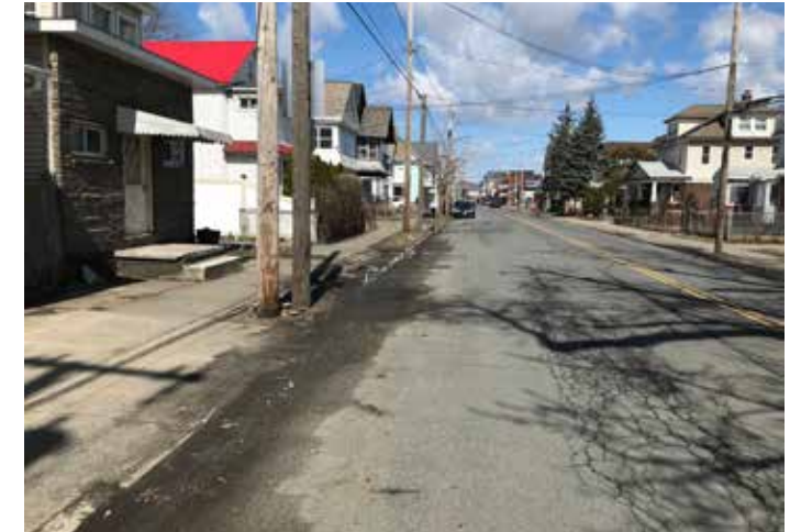
Drainage is challenging and problematic in areas like this one between Main Avenue and Ostrander Place where the road is higher than the edge of sidewalk and there is no curb reveal. This photo was taken between Main Avenue and Ostrander Place.
