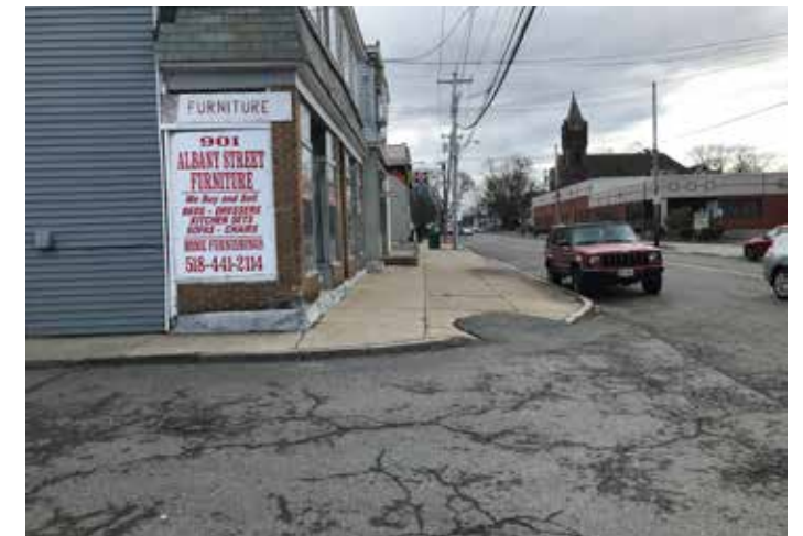
Several intersections are lacking in ADA curb ramps and crosswalk striping. This photo was taken between Steuben Street and Craig Street.
