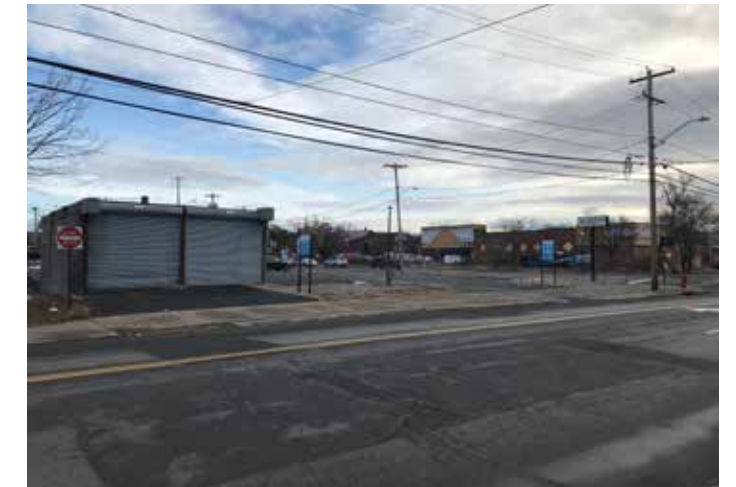
There is no sense of a street wall at this highly visible and important northern corner of Albany Street and Brandywine Avenue where the lot is occupied by parking and contains no street trees. This situation likely contributes to higher speeds on Albany Street. The absence of trees also calls greater attention to the unsightly overhead utility lines,
