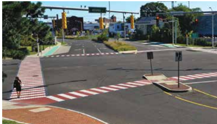
Decorative Crosswalks can help emphasize the presence and importance of pedestrian crossings. Image Credit: The Who's Who in Building & Construction, Rocco Iadarola General Contracting Company
