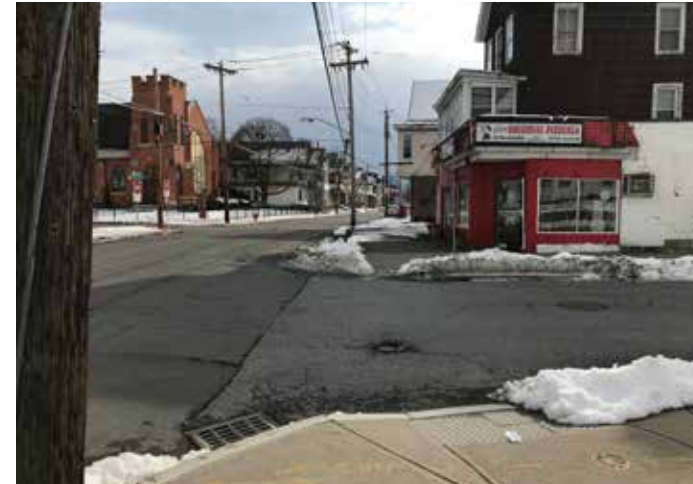
Some ADA curb ramps have been added, but many intersections lack crosswalk striping. This photo was taken between Main Avenue and Ostrander Place.
