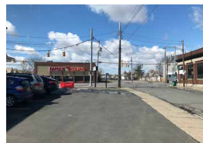
The parking lot at the Crane / Main / Chrysler intersection has a low to zero curb reveal, which functions as a 170' curb cut and encourages cars to back into the road at points very close to the intersection. It is also lacking in any vertical elements that could help with traffic calming and enhancing the pedestrian experience.
