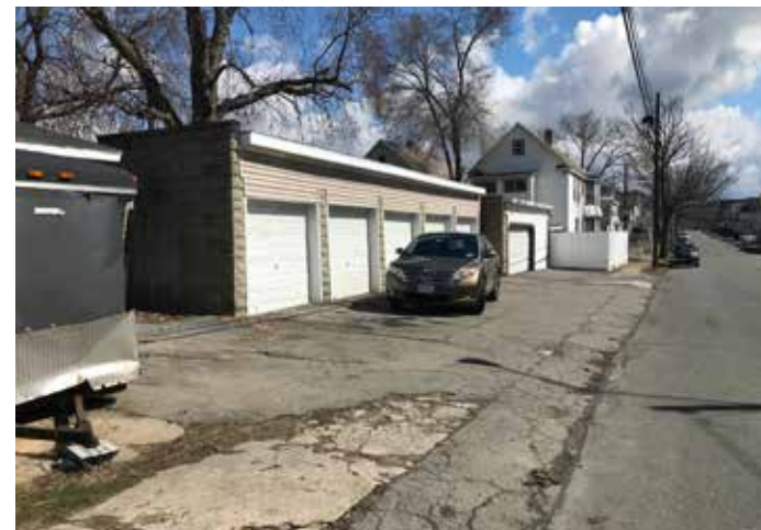
Portions of the sidewalk have been paved over with asphalt. In the instance above, this long garage prohibits on-street parking and preferences vehicular use over pedestrian travel.
