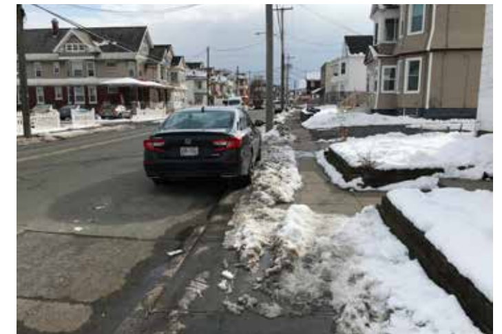
Parking on the sidewalks happens even more frequently during snow events. This photo was taken between Main Avenue and Ostrander Place.
