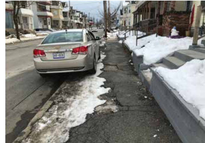
Many sections of Crane Street include sidewalks that have been paved over with asphalt, as well as cars that frequently park in the sidewalk zone, making use of the sidewalk difficult, if not impossible. This photo was taken just south of Ostrander Place, but illustrates a common condition along Crane Street.
