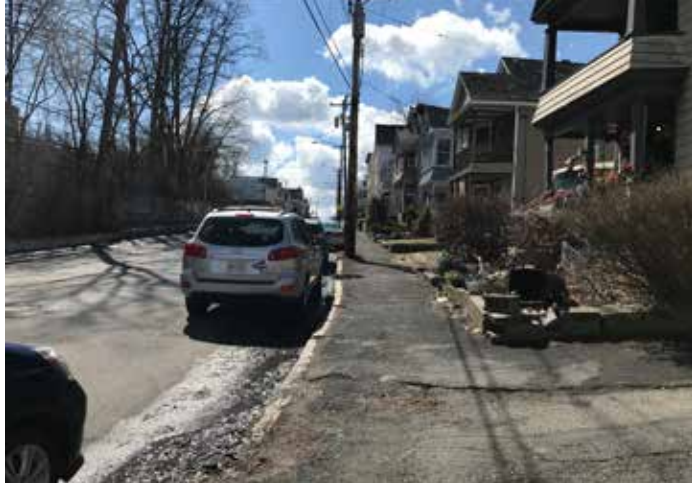
Large sections of sidewalk have been replaced with asphalt between Bridge Street and Broadway. The sidewalk is also very narrow in several places where utility poles exist and there are no street trees on the west side.
