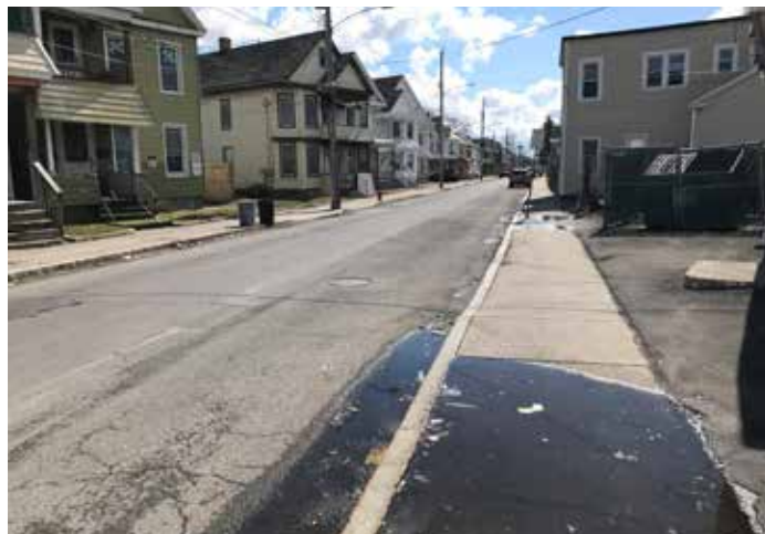
Several sections of sidewalk along Chrisler Avenue have ponding issues. Parking during the day is fairly minimal. The road is also narrow for a two lane road with one aisle of parking and there are almost no street trees.
