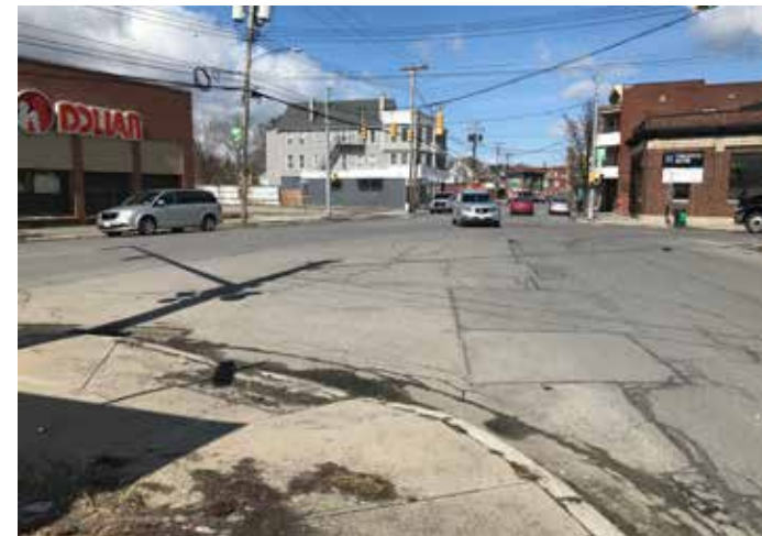
There is an ADA access ramp at the point of the property between Crane and Chrysler, but it leads to the center of the intersection, encourages maximum length and exposure crossings, and there is no crosswalk striping at the intersection.
