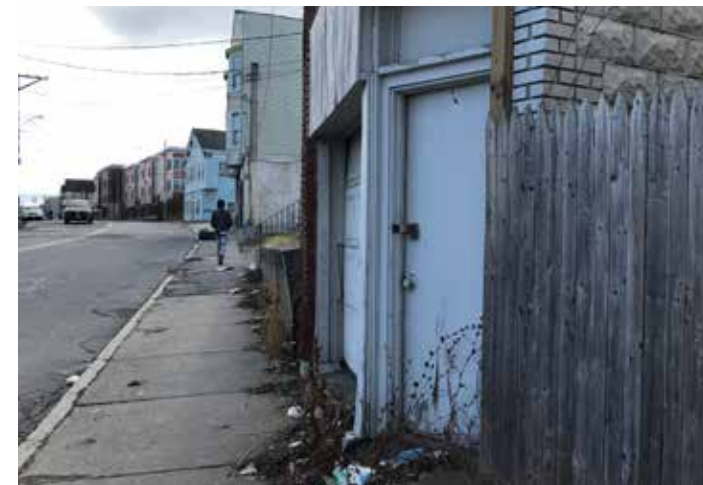
This section of sidewalk on the west side of Albany Street between Paige Street and Veeder Avenue illustrates the challenges posed by narrow sidewalks, topography, and excess litter along the corridor.
