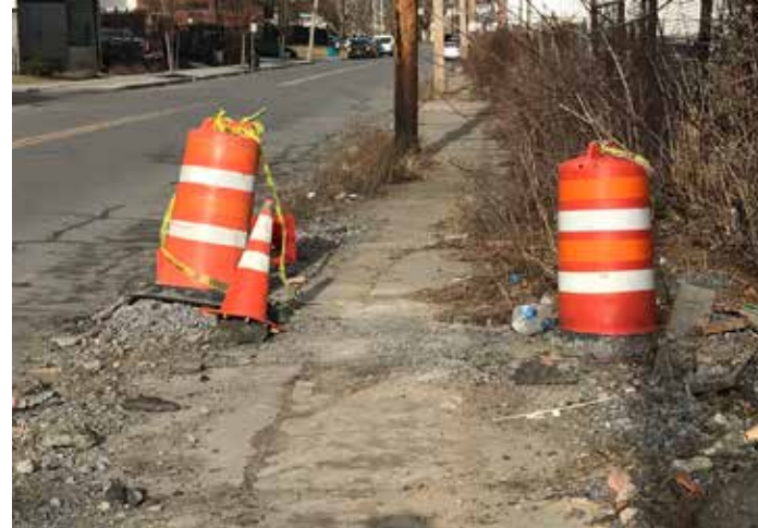
Many areas that occur along the “back yards” of businesses that front on State Street are missing sidewalks and have become impassable. This photo was taken between Craig Street and Veeder Avenue.
