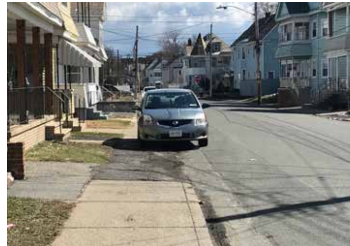
Main Avenue is narrow in the section between Crane Street and Willett Street and cars frequently park on and obstruct the public sidewalk.
