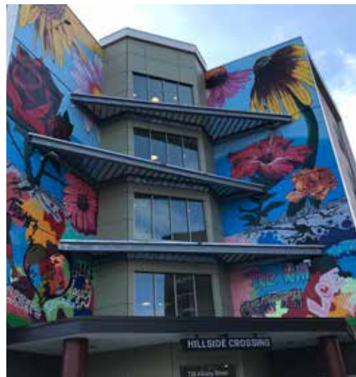
The "Best Kept Secret" gateway mural on the Hillside Crossings building on Albany Street was painted in 2021 by local artists Rae Frasier and Eugene O'Neill.
