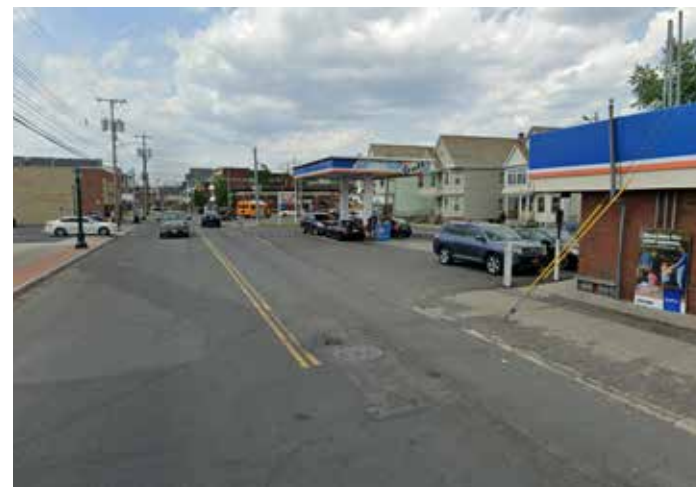
The sidewalk on the east side of Crane is missing in the south area closest to the Main / Crane / Chrysler intersection, which makes walking more challenging, encourages higher speeds, and adds to the general confusion in the area of the intersection..
