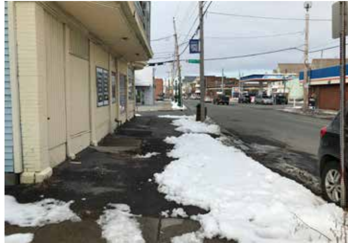
Many areas of sidewalk have been paved over with asphalt as shown here at the 6th Avenue intersection.
