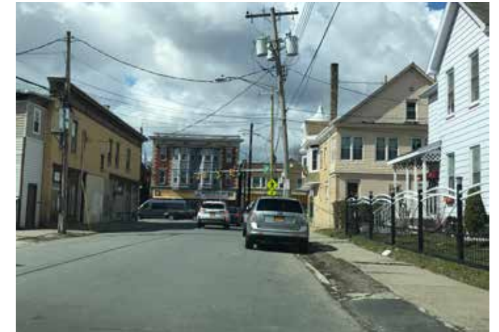
Cars frequently straddle the curb on Francis Avenue. In many locations, the road is higher than the curb and the tree lawn fills with ponding during storm events. As seen in this photo, the area that should be filled with grass has been severely compacted and is now a low spot.
