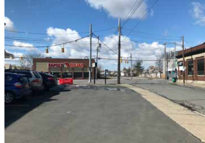
The sidewalk closest to the Crane / Main / Chrysler intersection doubles as a vehicular use area where there is no curb reveal and cars back over it to enter and exit the parking area.
